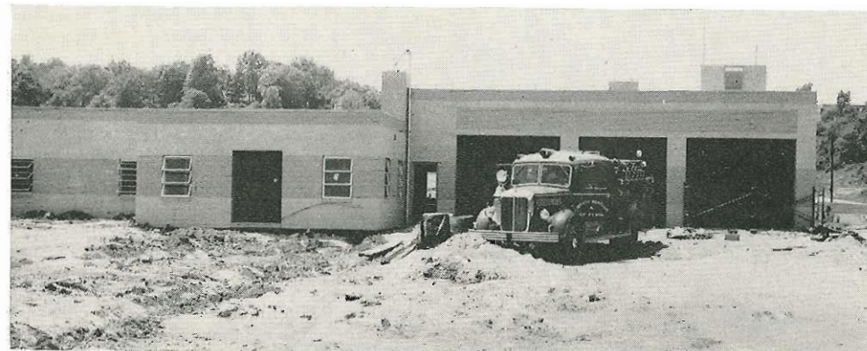
NEW FIRE HALL BEING ERECTED IN LIBERTY BORO
